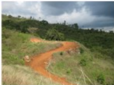
Stan's driveway ready for rock
