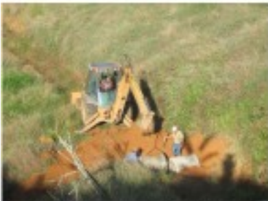
Installing culverst in Stan's driveway in March 2011
